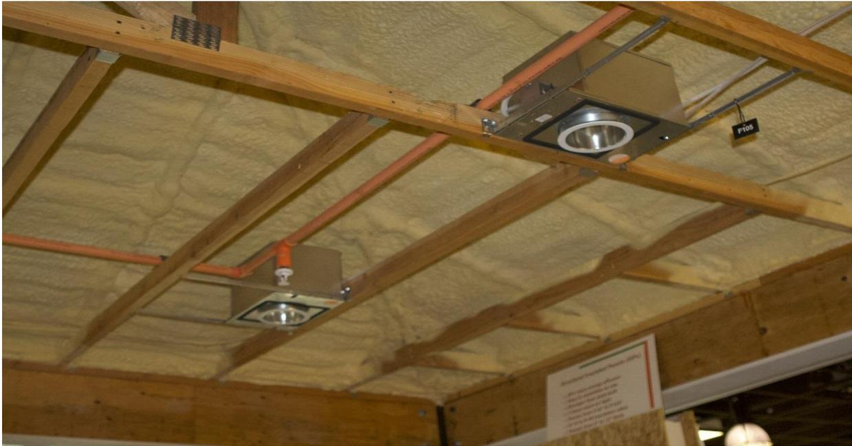
*Figure 4: The recessed lights in attic floor of this unvented attic construction didn't need to be made airtight. By not performing such airtightness measures construction costs savings can be realized even if no HVAC equipment and ductwork are located in the attic – a situation common for many cold climate locations. Image Courtesy of Icynene Inc.*
