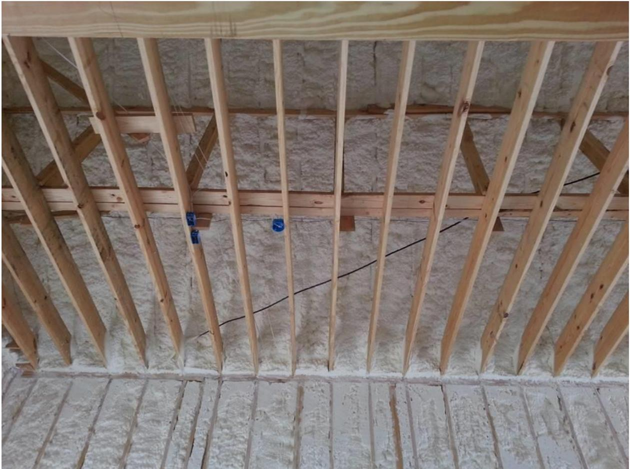
*Figure 2: Looking upward through the open ceiling, if the exterior wall and roof deck assemblies both contain spray foam then a continuous insulation and airtight layer is established from the base of the walls to the peak of the roof. A very energy efficient enclosure results. Image Courtesy of D7 Spray Foam Insulation, Houston TX*
