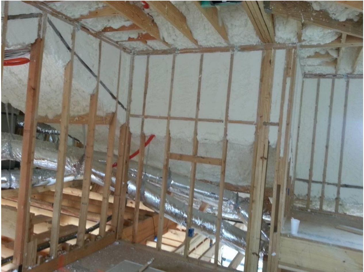
Figure 1: Instead of insulating and making airtight walls adjacent to a vented attic space an unvented attic application using spray foam eliminates this need in this difficult to access assembly. Image Courtesy of D7 Spray Foam Insulation, Houston TX
