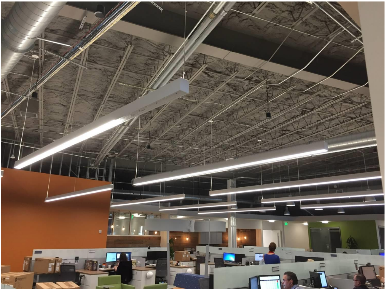
Figure 3: Gaining in popularity is the design approach of insulating on the underside of the roof deck and leaving the spray foam exposed to the occupants below. This variation on the unvented attic design requires a thermal barrier, such as an approved intumescent coating. As shown in this workplace setting, painting of the foam is possible to make it less obvious. Image Courtesy of Icynene Inc.
